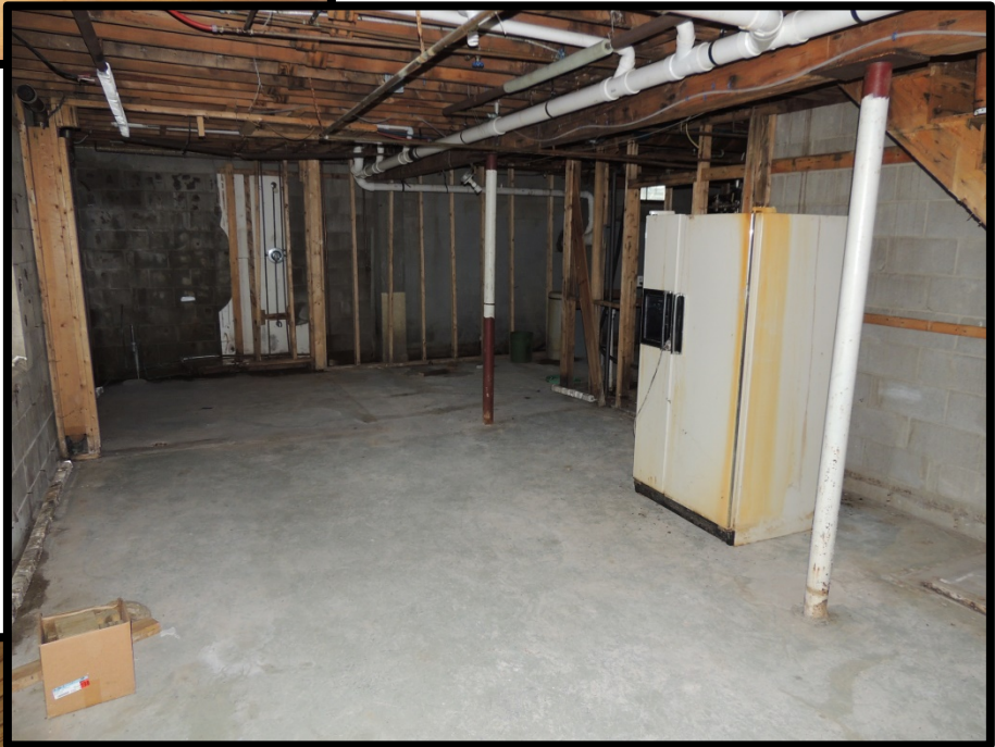
Large Unfinished Basement
